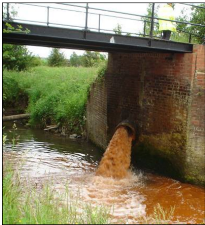
Figure 1. Point source: Kibblesworth coal mine water discharge before it was remediated.
